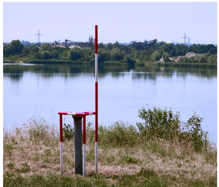
Figure 3 - The groundwater monitoring well shown in this photo is a common component of remedial activities.
